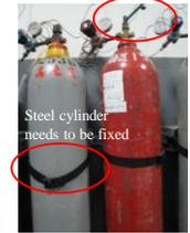
Spare cylinder and empty cylinder should be furnished with cap
